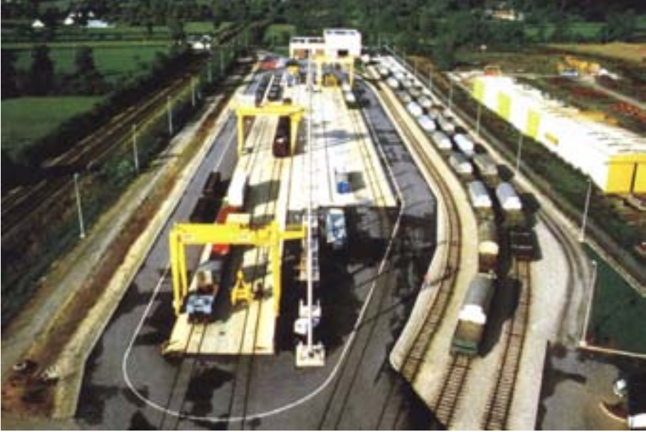
FIG. 11. The COGEMA Logistics rail to road trans-shipment terminal in Valognes.
