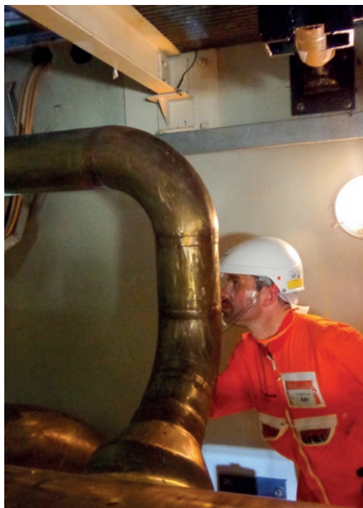
Hydrotesting of the primary system of reactor 4 in the Cruas-Meyssse NPP, May 2016.
