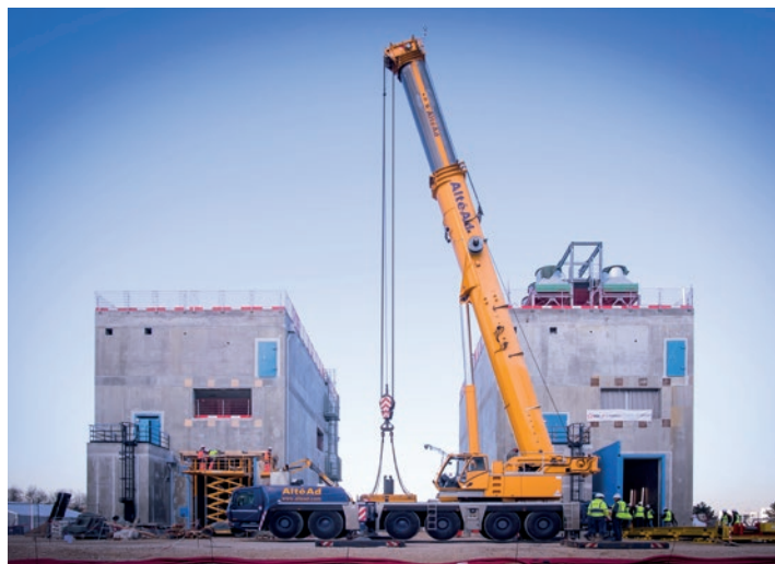
Installation of an ultimate back-up diesel generator on the Saint-Laurent-des-Eaux NPP, November 2016.
