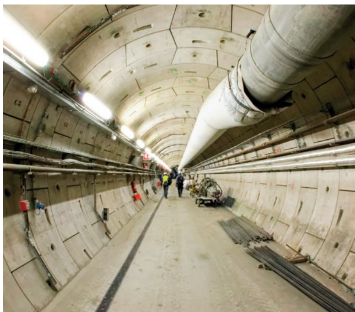
Underground laboratory of Meuse/Haute-Marne: rigid design drift.
