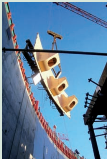
Installation of support brackets on the inner containment wall of the Flamanville 3 EPR reactor building
