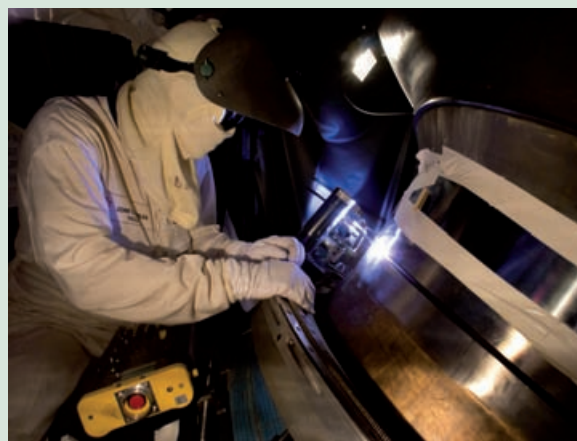
Tig Orbital Narrow Gap welding operation: connection of the steam generator to the reactor cooling piping on the hot leg side
