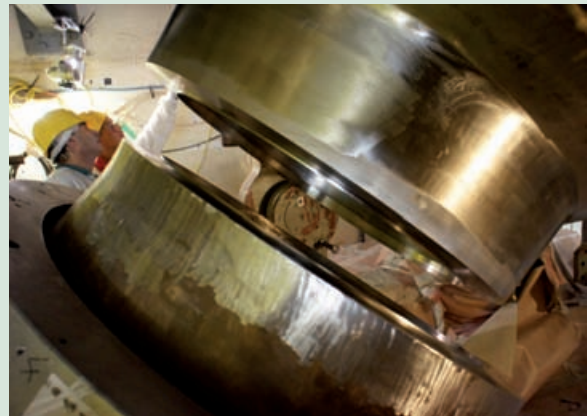
Mating of the steam generator with the reactor cooling piping on the hot leg side
