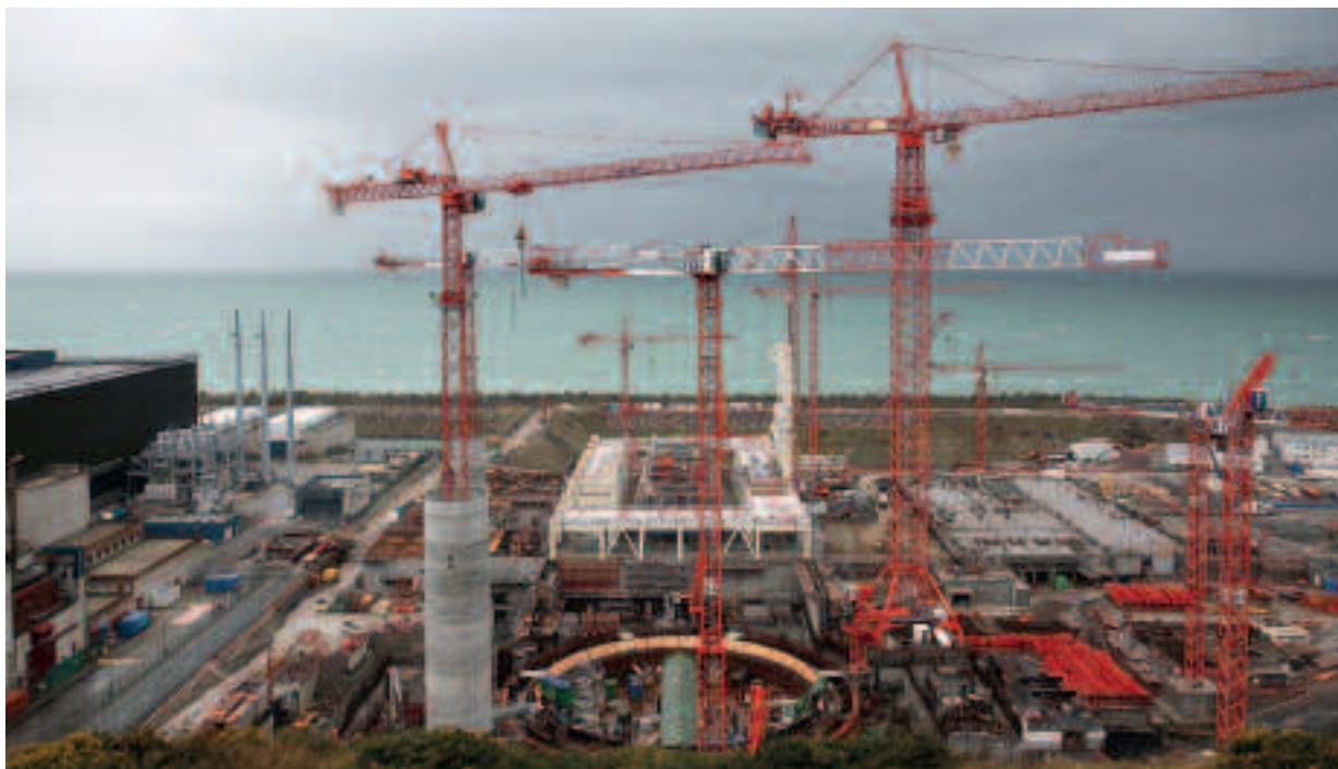
General view of the future EPR Flammanville 3 reactor (Manche département) – January 2009
