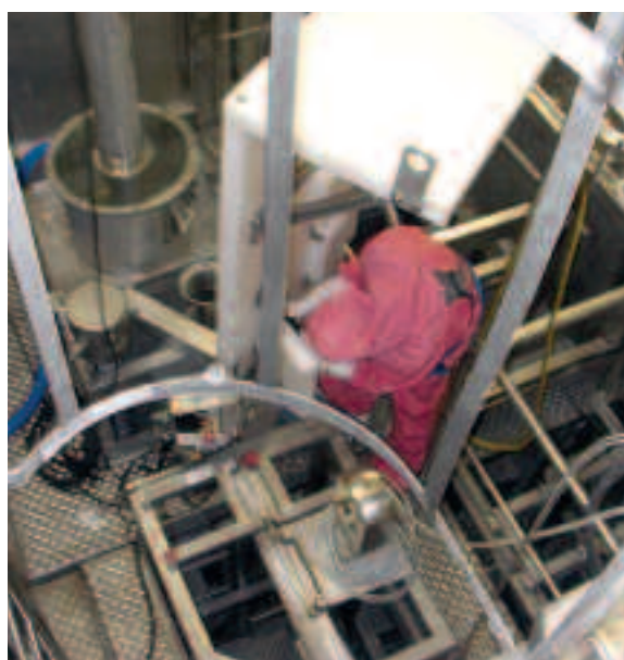
The HAO facility at La Hague during decommissioning in 2007 (Manche département)
