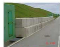
Consolidation of slope
