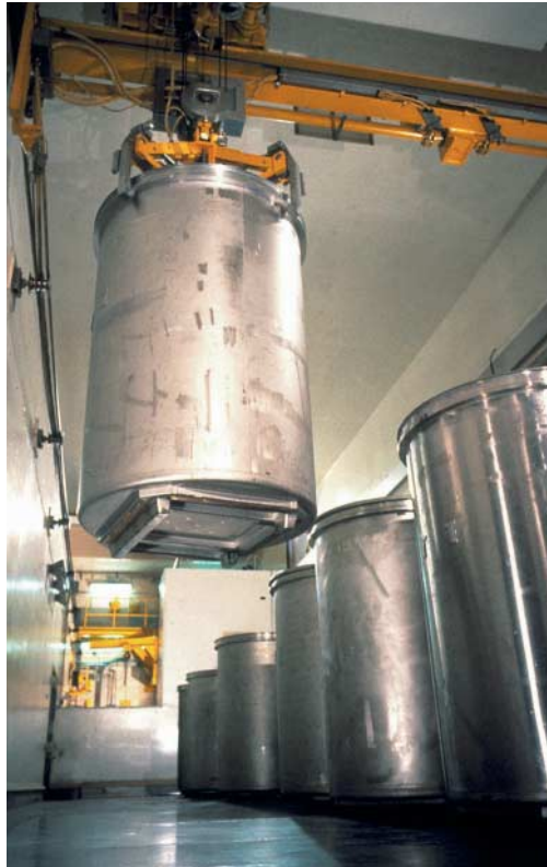
Handling of casks containing cemented hulls and end-pieces in the storage hall at COGEMA's UP3 plant in La Hague
