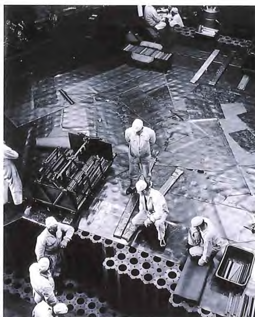
Graphite stack in a gas-graphite Uranium reactor
