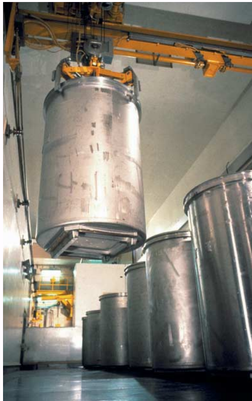
Handling of casks containing cemented hulls and end-pieces in the storage hall at COGEMA's UP3 plant in La Hague
