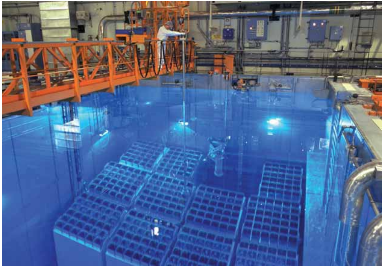
Racks in Bk pool comprised of cells for storing spent fuel
