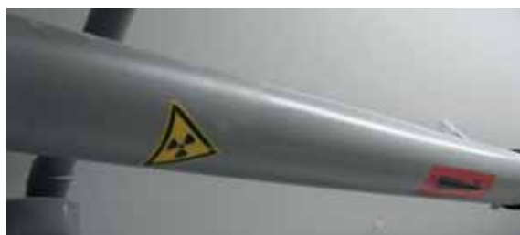
Pipes carrying contaminated liquid effluents
