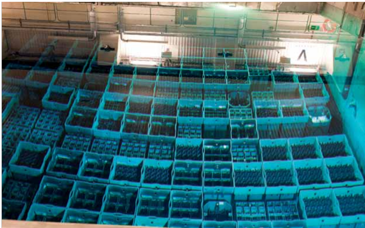
Subsurface (-25 meters) storage pool for spent fuel in granite. IRSN visit to the facilities of the Swedish waste manager, SKB
