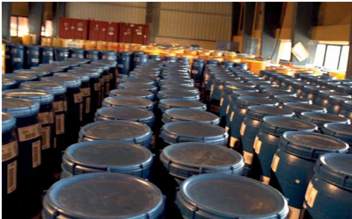
Dismantling of the nuclear power plant EL4 at Brennilis - storage of radioactive waste
