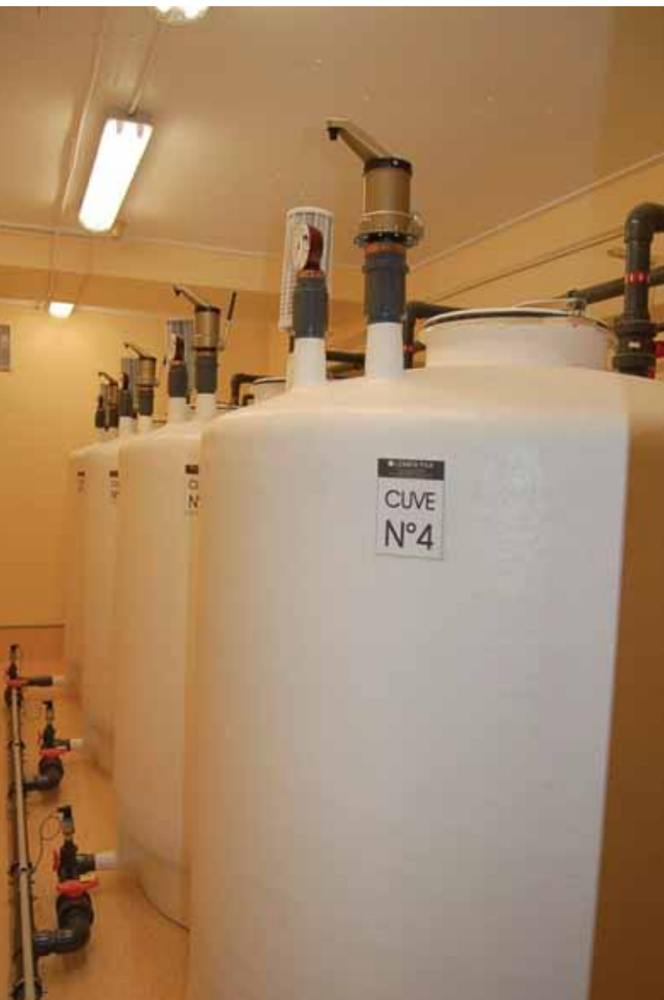
Storage tanks for contaminated liquid effluents from a nuclear medicine department
