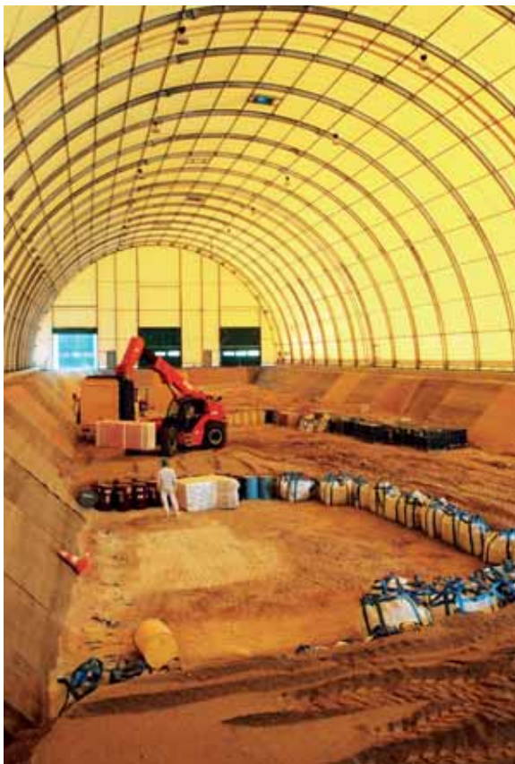
Placing VLLW (very low-level waste) in “big bags” into a disposal cell which was excavated a few meters deep into the clay rock
