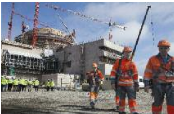
IRSN visit to the EPR construction site at Olkiluoto in Finland. Workers, cranes and reactor building with the containment dome designed to withstand an aircraft crash
