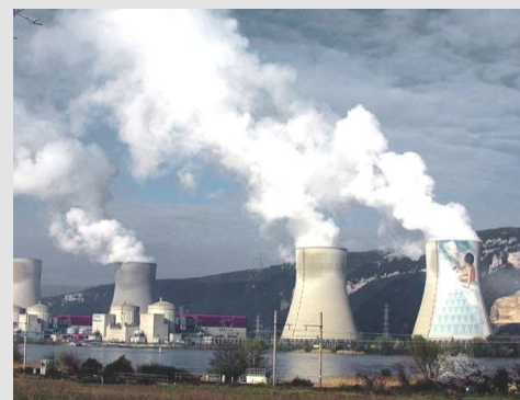
The Cruas-Meysses NPP
